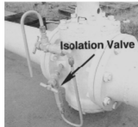
MANUAL BLEED WITH THERMAL RELIEF (MTR)
