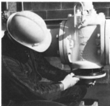
LOWER PLATE REMOVAL
