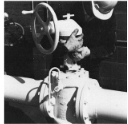
OPERATOR REMOVAL
