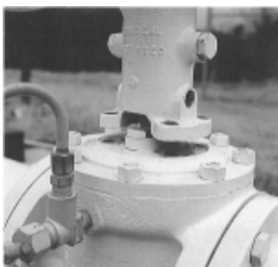
PACKING GLAND BOLTS EXPOSED
