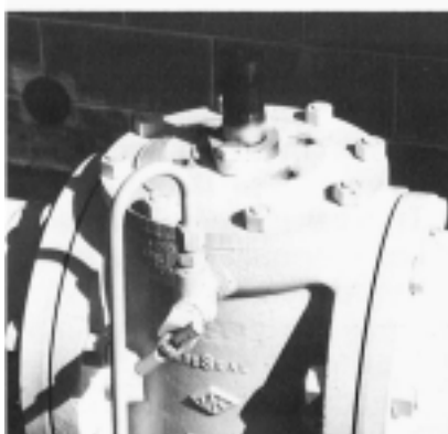
VALVE WITH OPERATOR REMOVED
